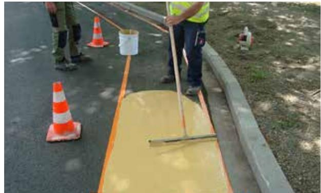
These are mainly coloured coatings, which may or may not be reflective, with very quick curing and a non-slip surface. The range also includes fast-curing adhesives to stick reflectors into the road.
