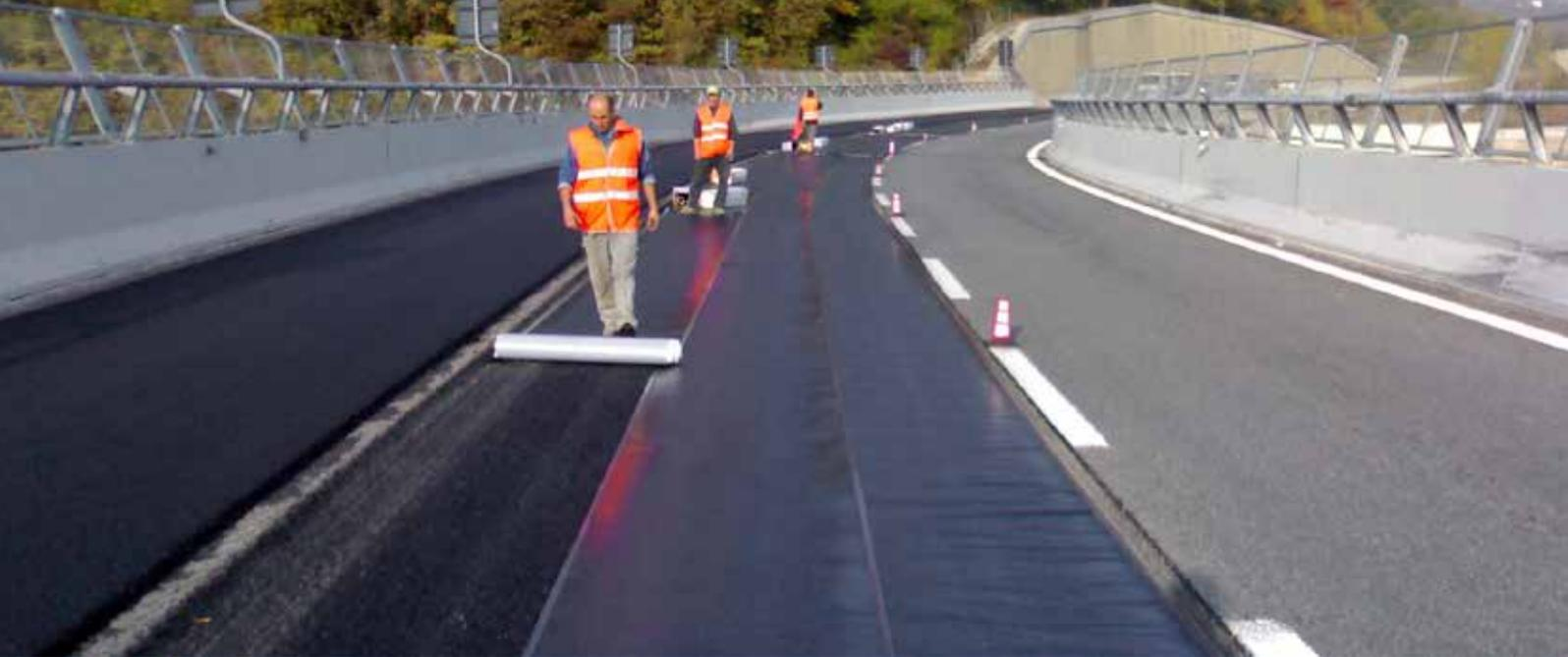
**IKO polybridge** is a waterproofing membrane composed of plastomer (APP) bitumen and a polyester-glass fibre composite reinforcement. The upper surface is finished with talc and the lower surface is covered with a thermofusible film. IKO polybridge, when combined with protection consisting of mastic asphalt or road asphalt, offers an adequate solution for car park roofs, bridge decks and tunnels with a bonded waterproofing system that can be operational immediately after installation.
