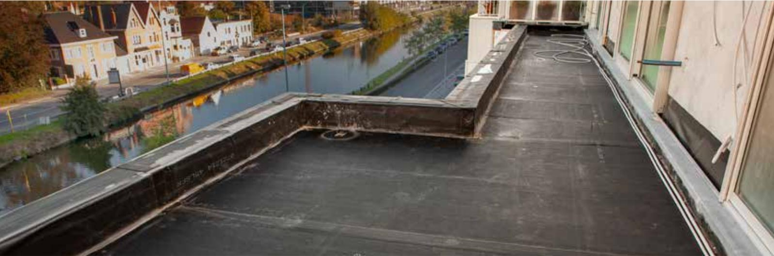
Besides the traditional flame welding of bitumen membranes, there are also many other ways to make a flat roof perfectly waterproof. When blowtorches are banned from the roof, roofers can apply the bitumen entirely without flame, using self-adhesive membranes, cold gluing or mechanically fixed systems. IKO offers the appropriate membrane or system for every one of these solutions. The overlaps in IKO roofing rolls can be welded with hot air or using an 'encapsulated flame'.
