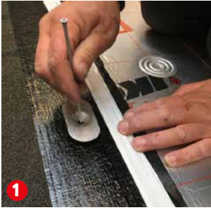
1 Mechanically fastening of underlay
